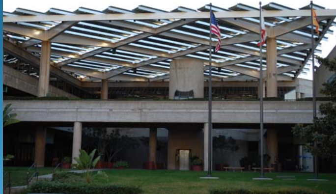
Utilized Existing Atrium Structure
